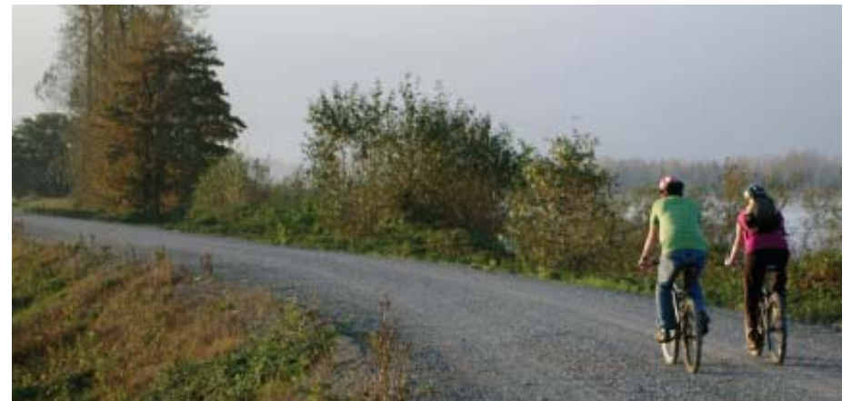
Fraser River East Dyke, Chilliwack
